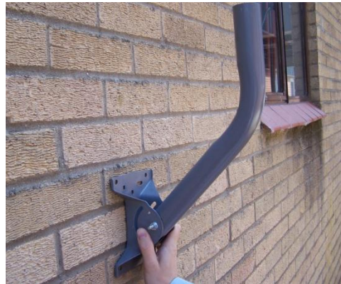
Figure 4-3 – Pole Assembly
