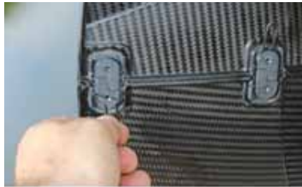
Figure 3-5: Latches to interconnect the panels
